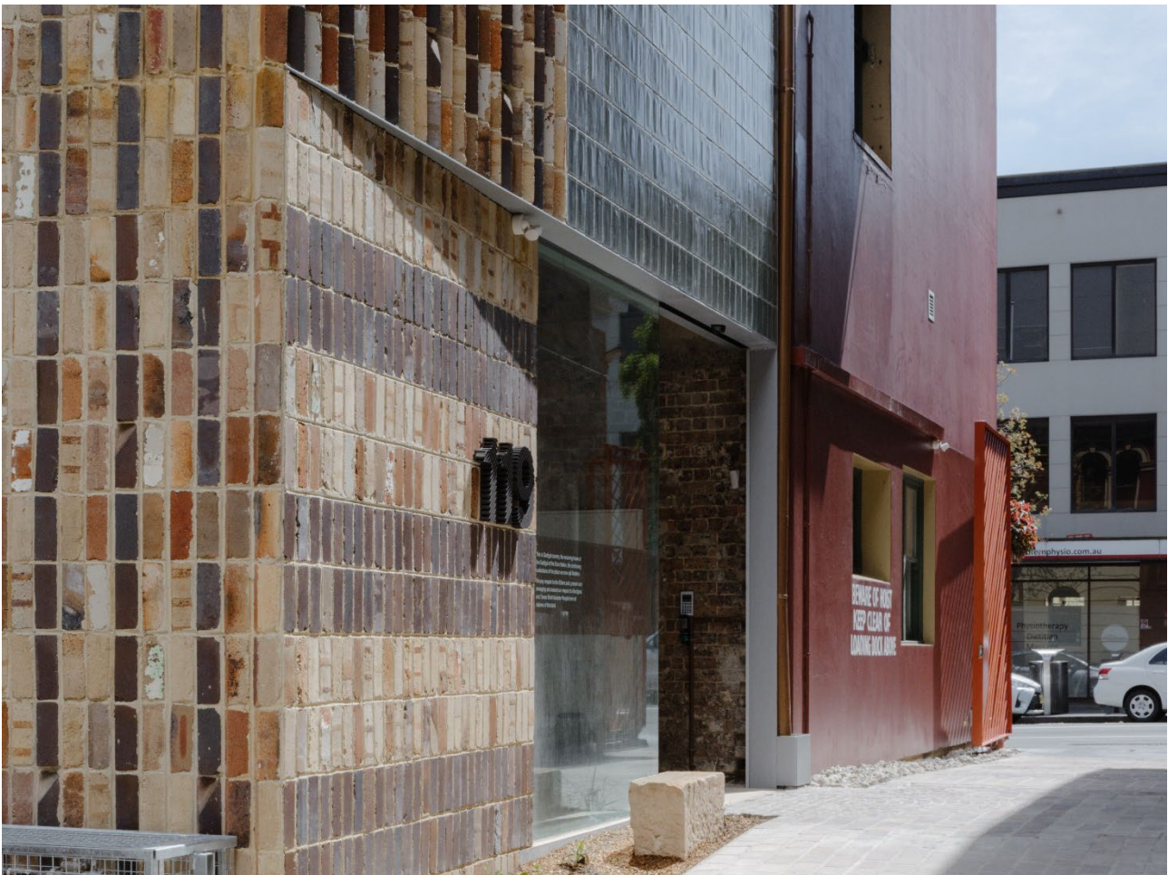
Reused brick façade at 119 Redfern (Photo by Aileen Sage / City of Sydney)
